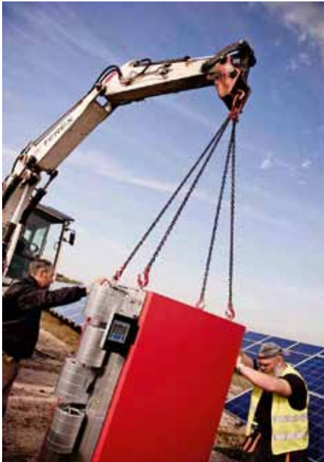
Installation of a central inverter
